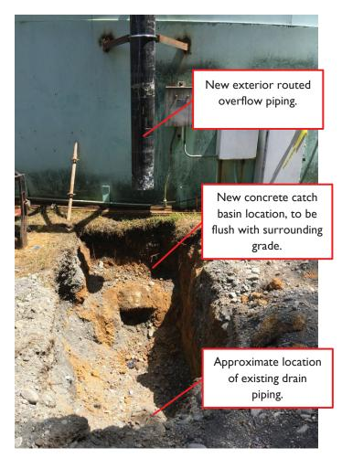
Figure I: Excavation for overflow drain catch basin.
