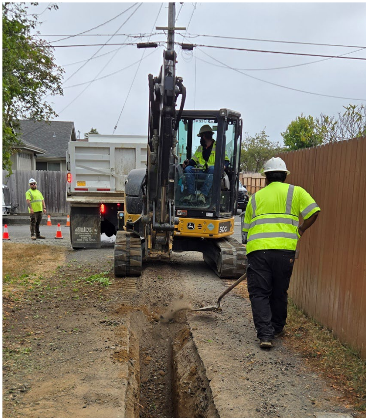
Figure 1: HCSD staff working on a steel main replacement CIP project on Shady Lane.
