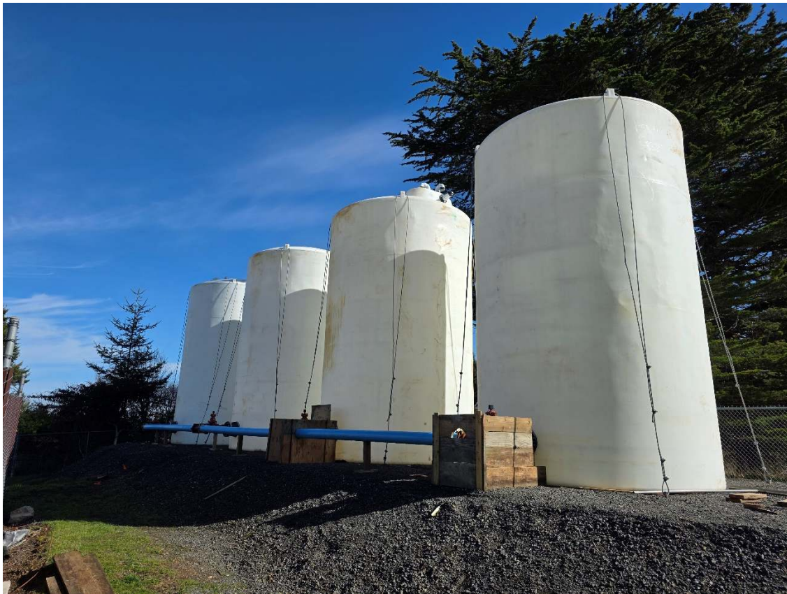
Figure 1: This picture shows the four recently installed temporary water storage tanks at the District's Donna Drive Water Tank Site.
