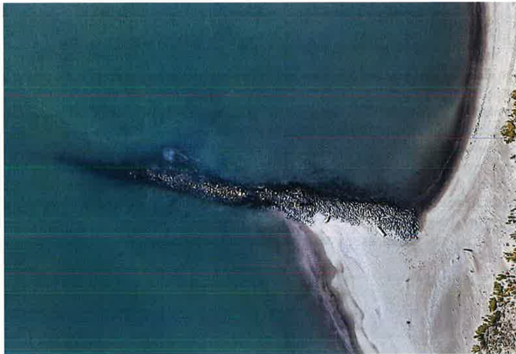
Figure 4 Erosion Observed at East End of Armor Stone (Google Earth, 2019)
