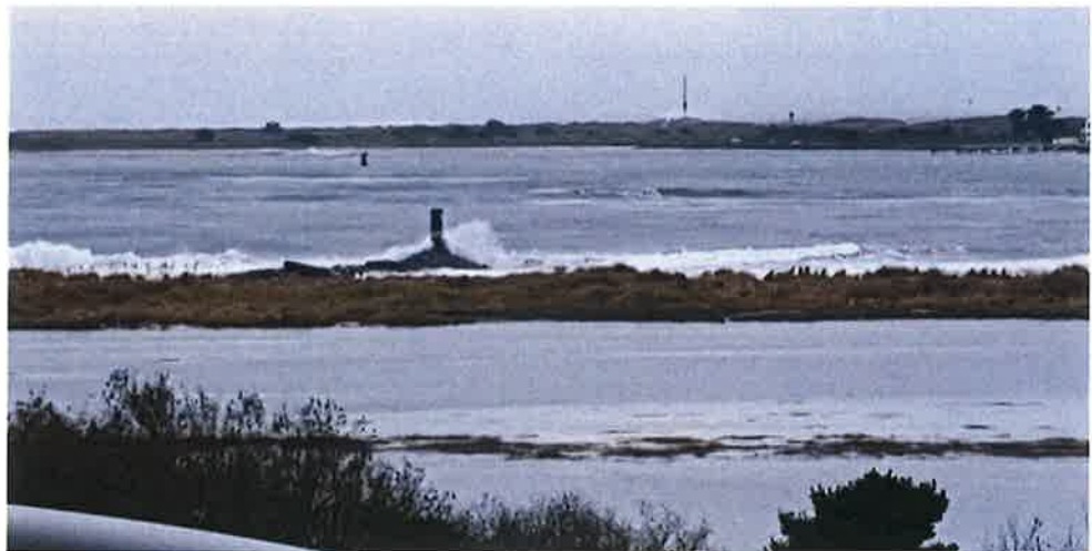
Figure 4: Standpipe on December 21, 2019 High Tide
