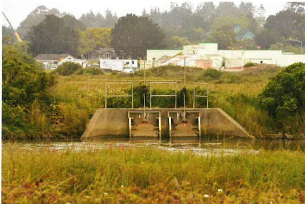
Figure 11: One of the Main Restoration Components in Area 1 is the Removal of Existing Tides Gates to Allow Tidal Inundation of the New Channel System. Removal of Barriers Such as this Will Increase Habitat for Fish and Aquatic Species
