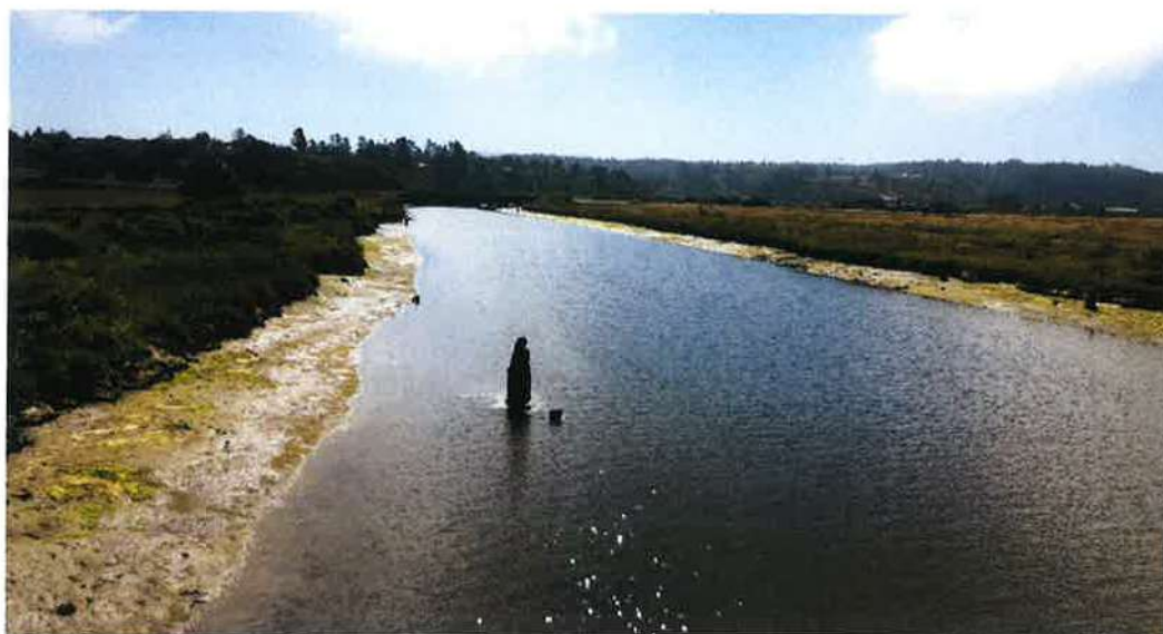
Figure 16: Looking East from Existing Bridge Crossing Elk River at Low Tide.
