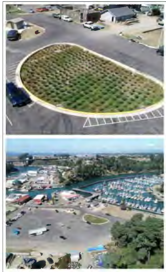
This photo presents a regraded and paved parking area with bioretention swale capturing and treating 100% of paved area runoff. The Noyo Harbor Boat Launch Facilities project was honored with a Merit Award from the American Council of Engineering Companies of California (ACEC).
