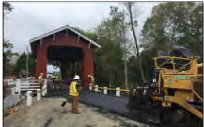
SHN provided construction management services for the County's Jacoby Creek Bridge rehabilitation.
