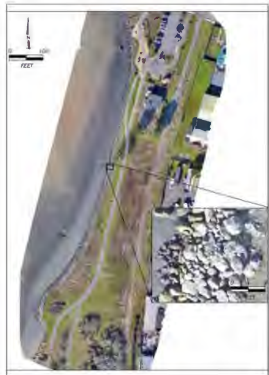
This image presents a UAV drone aerial from a flight over the City of Eureka's Hikshari' Trail.
