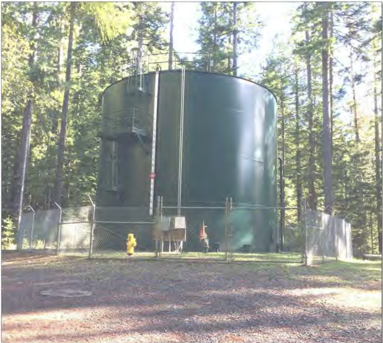
SHN was the project engineer for the City of Arcata's Upper California tank (welded steel).
