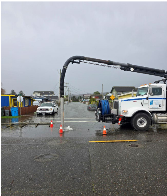
Figure 2: District Vac-Truck getting positioned to relieve the spilling manhole after tide recession
