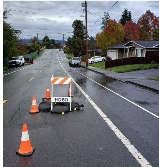
Figure 3: Manhole on Park sandbagged and coned off
