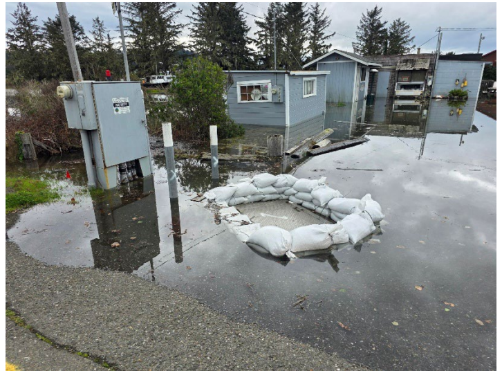
Figure 3: Sand bags surrounding King Salmon Lift Station to prevent further inflow and infiltration into the sewer system during high tide event
