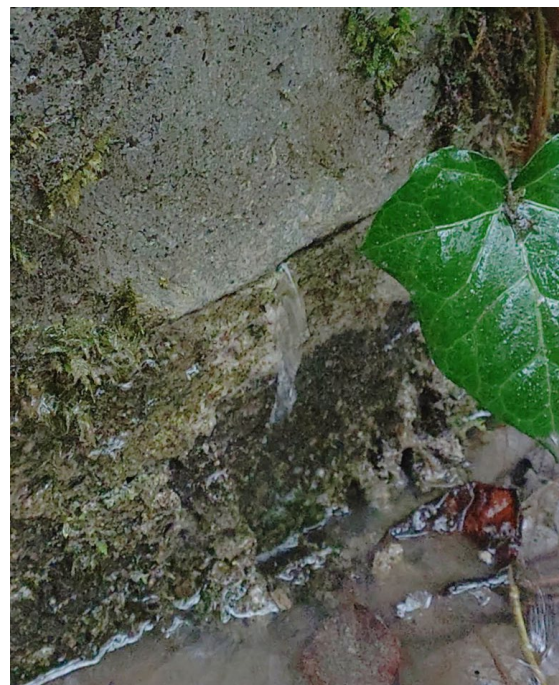
Figure 4: Sewer Escaping Manhole on North
