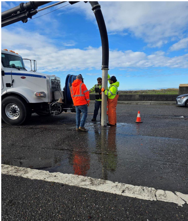
Figure 1: District Crews working to relieve the spilling manhole
