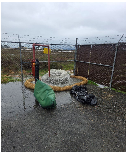
Figure 2: Sewer escaping the system at the Manhole at Hoover Lift Station
