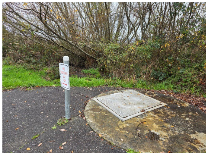
Figure 2: Edgewood Sewer Lift Station Well that overflowed
