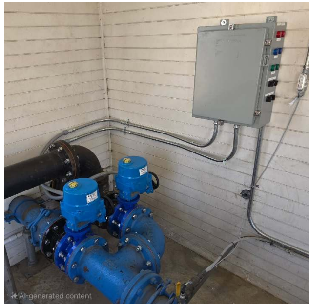
Figure 2: The photograph shows the newly installed automated butterfly valves used to remotely control which source the Hubbard Booster Station draws from.
