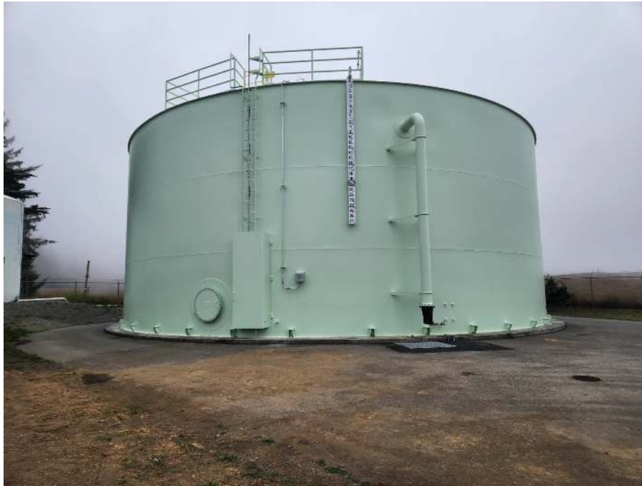
Figure 1: The photograph shows the rehabilitated 0.5 million-gallon Donna Drive Water Storage Tank. Upgrades visible include the new exterior overflow system, a liquid level indicator for improved monitoring, and a modern exterior safety climb system to meet current safety standards.
