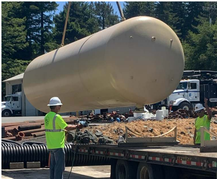
Figure 1: The new hydro-pneumatic tank being loaded onto a truck at the District's corporation yard.
