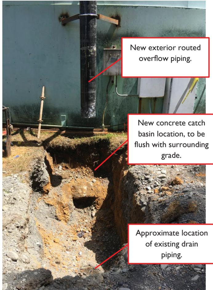
Figure 1: Excavation for overflow drain catch basin.
